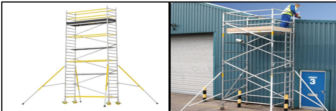
Figure 1: Example of a Scaffold Towers used for maintenance
